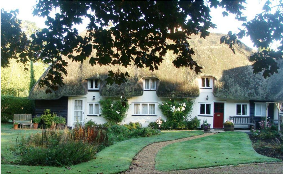
Picture 2: Patmore Cottage dating from the 17th century – one of a number of listed buildings in the settlement which are thatched
