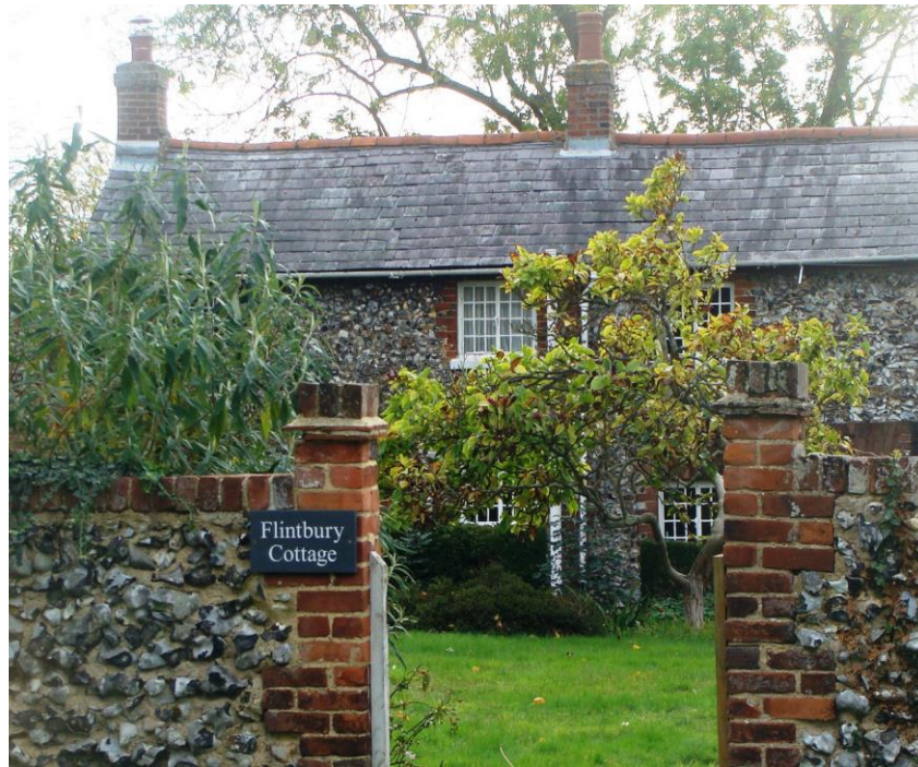
Picture 6: Flintbury Cottage, a charming 19 th century cottage of flint wall and slate roof construction. Boundary wall also included in listing
